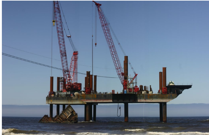
Barge with cranes held aloft on jacks.
